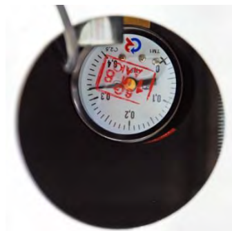
Fig. 2.7 Manometer installed at the bottom of the Primary Conversion Unit
